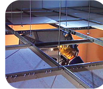
Position the unit in the suspended ceiling and fix it to the ties.
