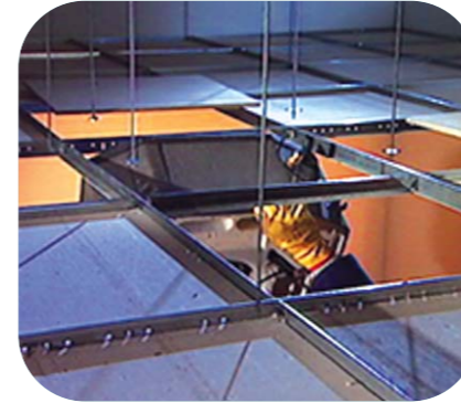
Fix the ties to the ceiling.
